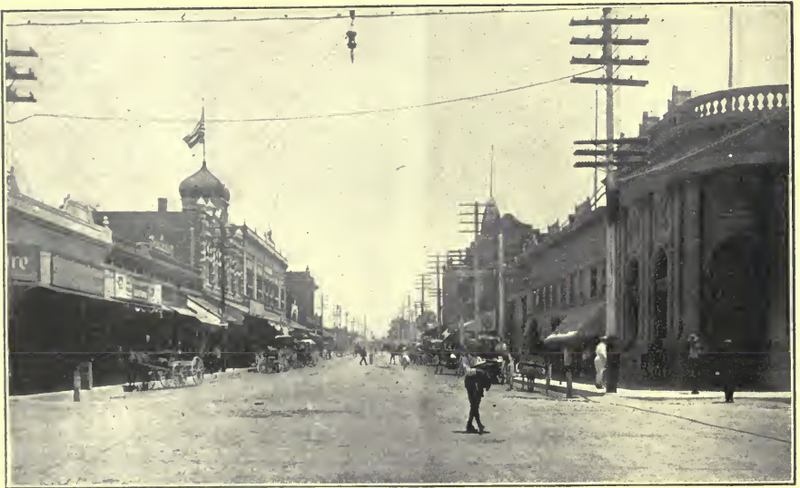
A TUCSON STREET SCENE.
